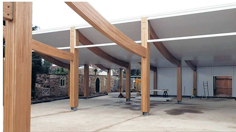
An innovative hardwood product for construction hybrid glulam based on spruce and oak (Picture HESS TIMBER GmbH & Co. KG).
