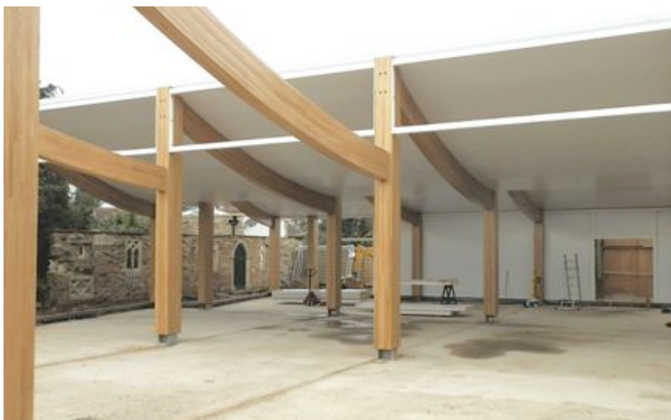
Hybrid glulam based on spruce and oak being used in the UK PHOTO: HESS TIMBER GMBH & CO KG
